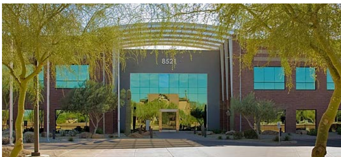
Scottsdale, Arizona Data Center located 30 minutes from downtown Phoenix.
